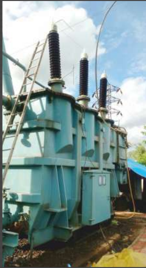
145 kV OIP bushings as Retrofit to old 145 kV SRBP bushings at an MPPTCL site
