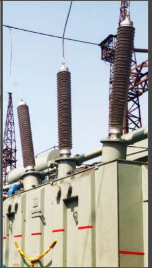
245 kV RIP bushing as Retrofit to damaged OIP bushing at JSW Dolvi
