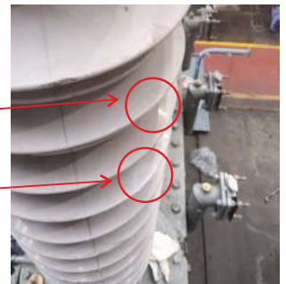
Repaired Silicone sheds on-site
