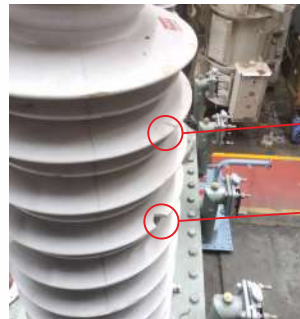
Damaged Silicone sheds at site
