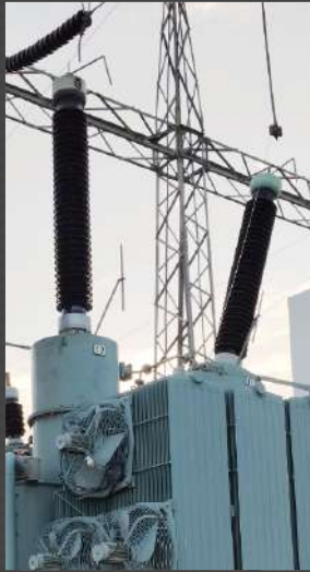
245 kV OIP bushing as Retrofit to damaged bushing of other manufacturer at an RDSO site
