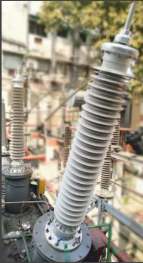
145 kV RIS bushing as Retrofit to old 145 kV OIP bushing at CESC
