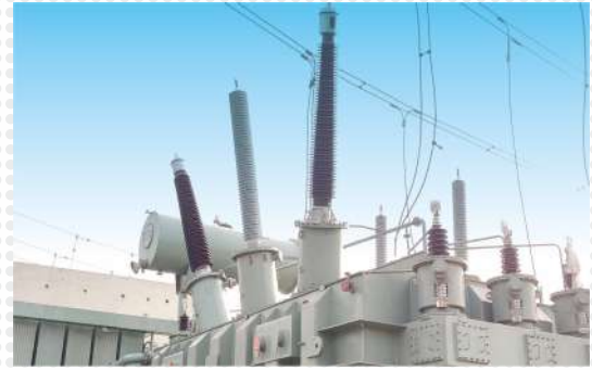
YASH® make 245 kV RIP bushing installed on a transformer as replacement to existing OIP bushing in Y phase, with R & B phase operating with old OIP bushings, at a site in Northern India.
