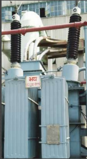
145 kV OIP bushing as Retrofit to damaged OIP bushing at Hindalco
