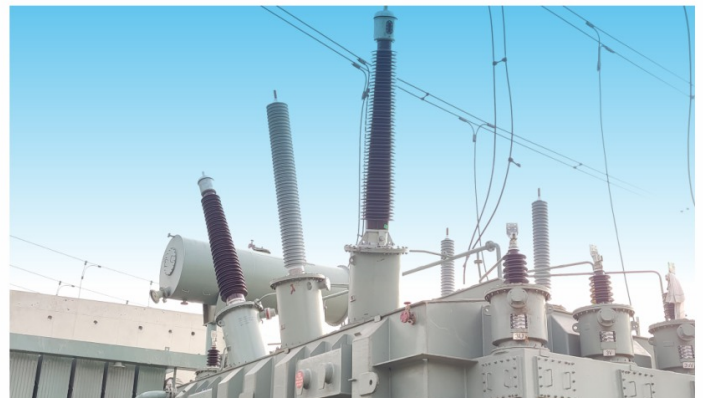
Y RIP Bushing installed on a transformer as a replacement to existing OIP bushing in Y phase with R&B phase operating with the old OIP bushings.
