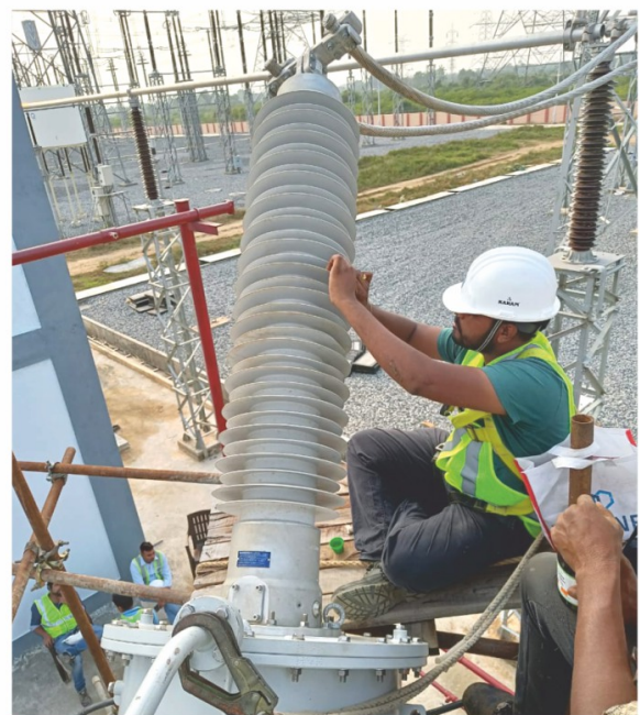
On-site Bushing repairing being carried out
