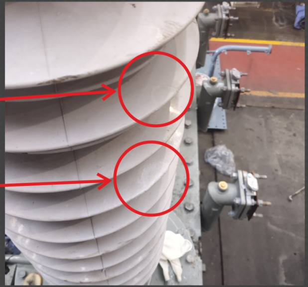
Repaired Silicone sheds on-site
