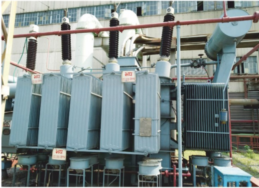
145 kV OIP bushing as Retrofit to damaged OIP Bushing at Hindalco
